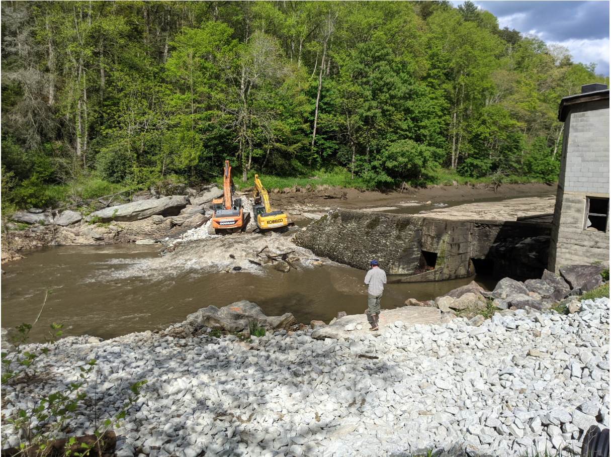
Figure 9: Image of the dam during removal showing downstream deposition of sediment burying the existing channel. Image credit to Josh Platt, 2021.
